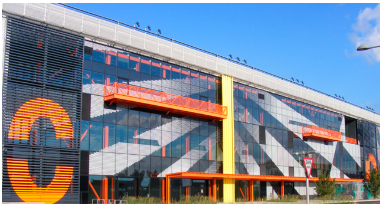
"Here East, former Olympic International Broadcast Centre" by Sludge G, licensed under the Creative Commons Attribution-Share Alike 2.0.
