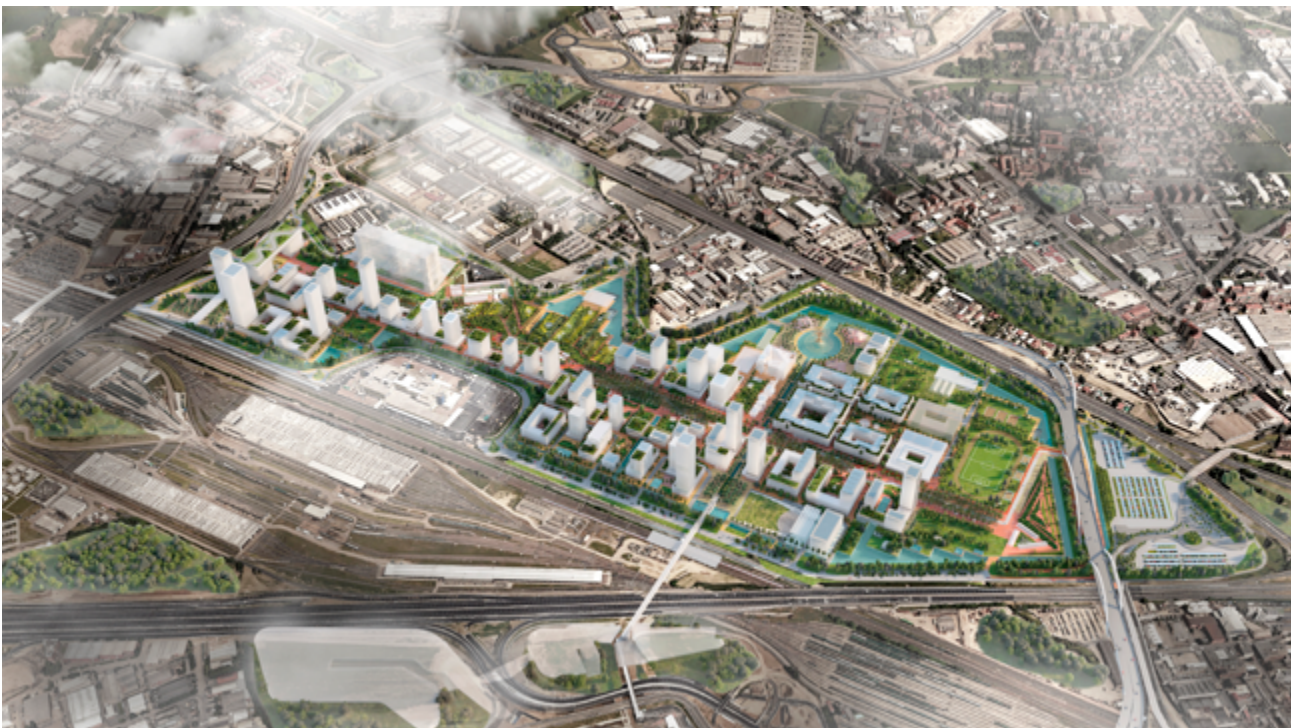
Figure 17. Milan Innovation District - MIND (in construction)
